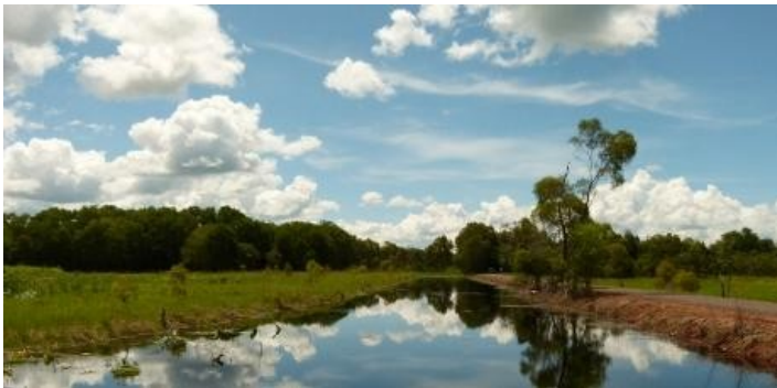
26 February 2012: view from lookout towards spillway
